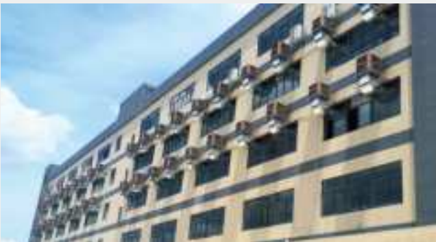
Home Appliance Factory
