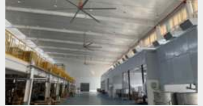
Powder Paint factory
