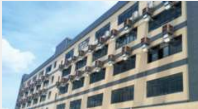
Home Appliance Factory
